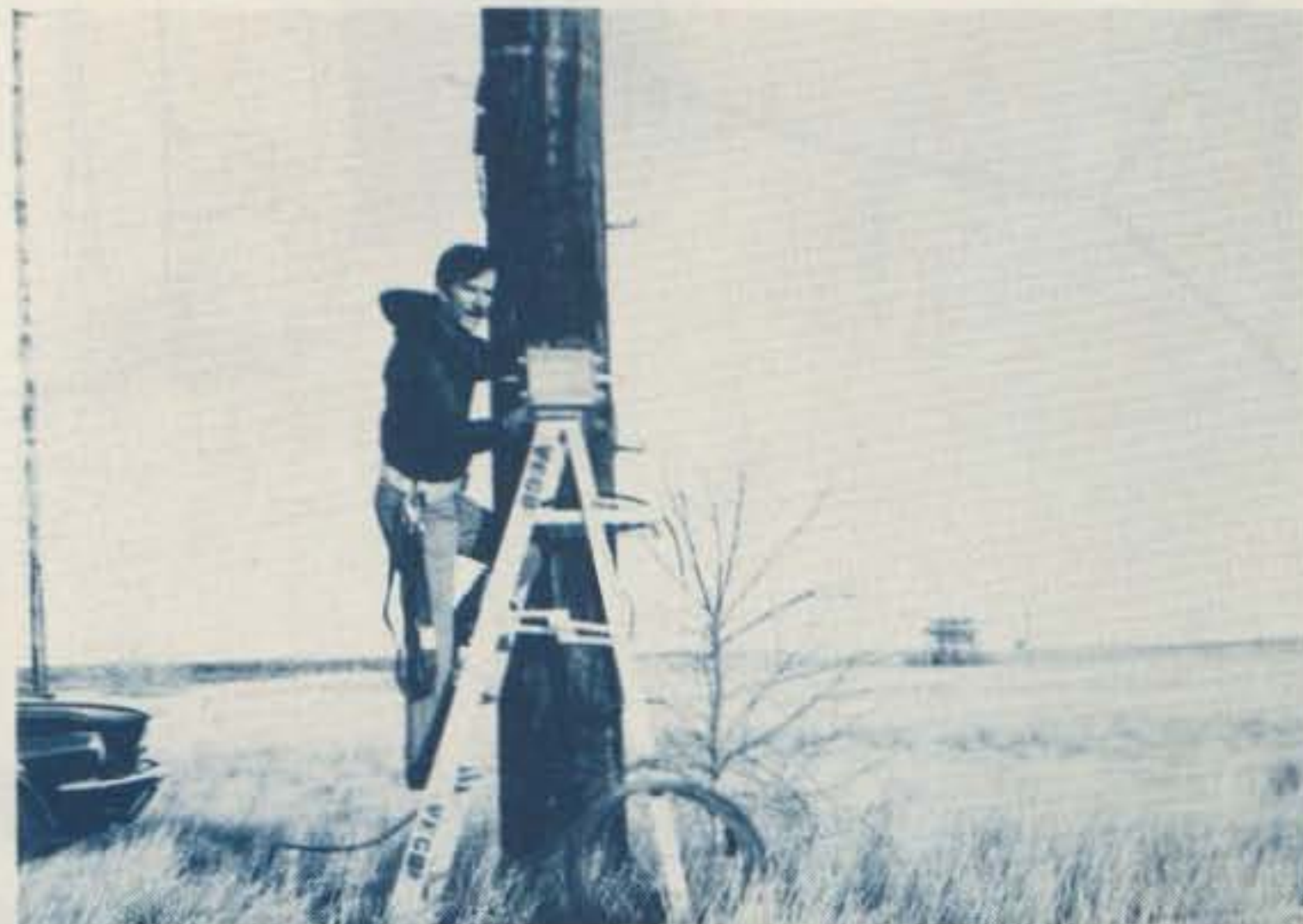
Installing the 1 kW broadband balun on the feed pole. The first two poles of my rhombic are used to support the beverage. The remaining poles are 20' long.
